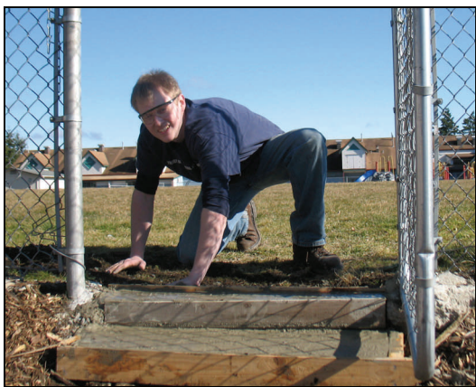
Hard at work building a concrete pad
